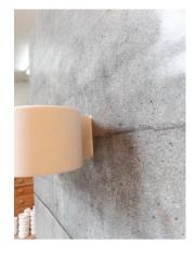
5. Once level use caulking to smoothen the interface between wall and light fitting.
