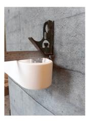
4. Gently press down on the light fitting until the light is level.
