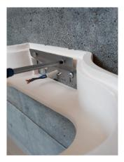
3. Secure light fitting in position over mounting bracket and tighten the two m4 screws against plaster until firmly secured.
