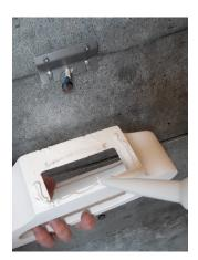
2. Run a bead of caulk around the lower area below and around cable entry opening. This prevents light spillage on uneven surfaces.
