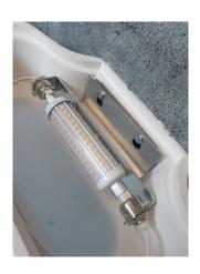
6. Insert lamp holder and connect wires.
